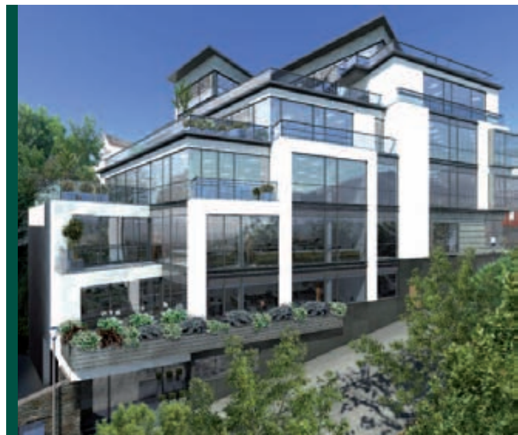
New offices at Finch Road
